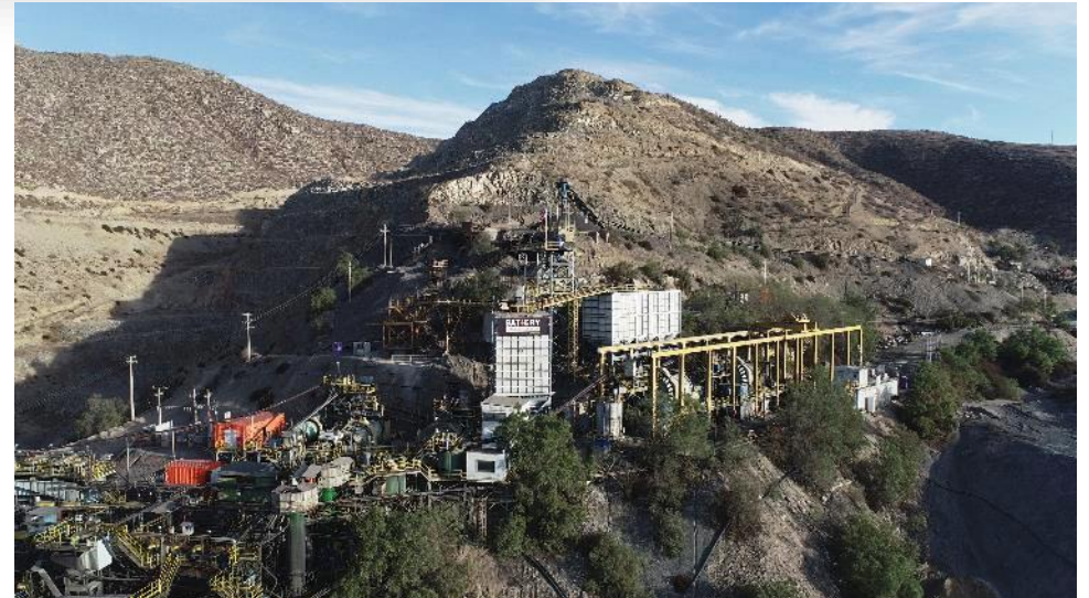
The Punitaqui Mining Complex, which includes the copper processing plant that is currently permitted for 100,000 tonnes per month
